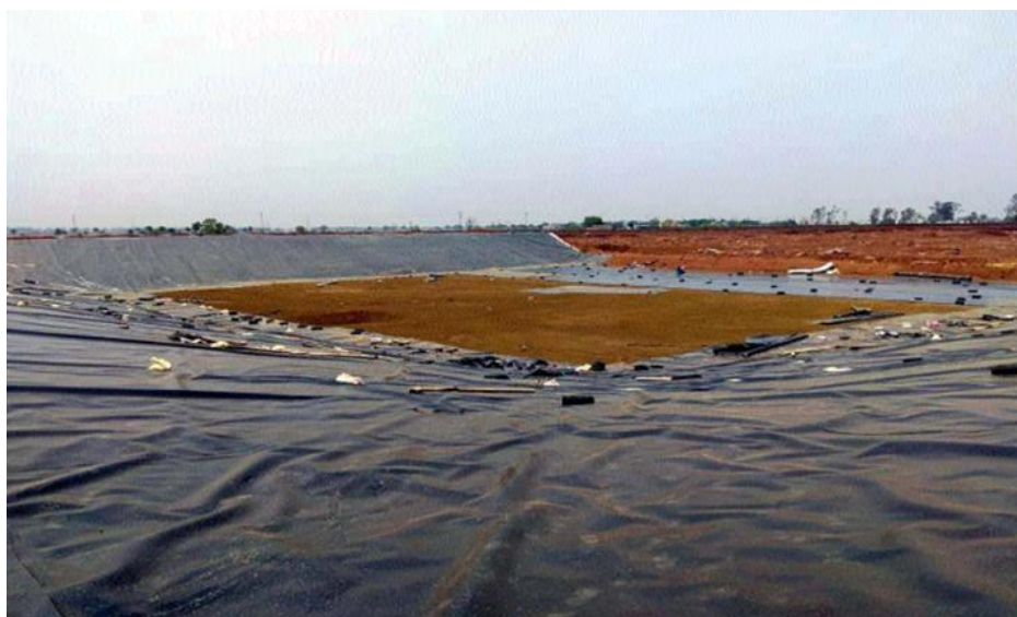
Figure 4.3: Sarona Trenching Ground at Siltara.
